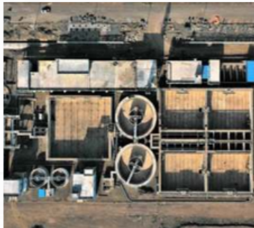
Common Effluent Treatment Plant 20 MLD Commissioned, expandable up to 60 MLD
