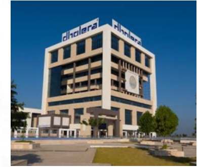
ABCD Building Administrative Building with City Integrated Operation Center
