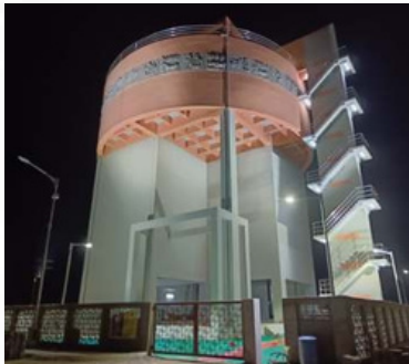
Water Supply & Storage Infrastructure 2 Master Balancing Reservoirs and 9 Elevated Service Reservoirs
